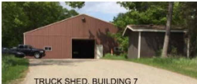
TRUCK SHED, BUILDING 7
