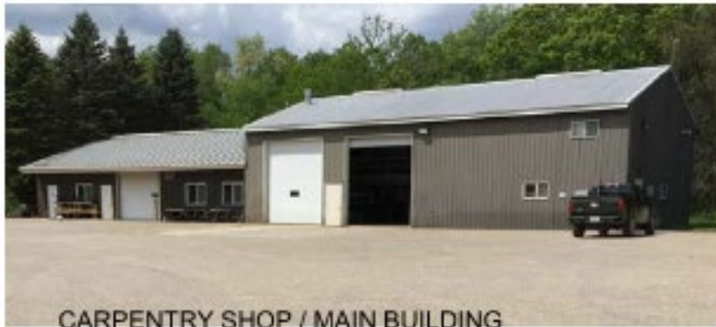
CARPENTRY SHOP / MAIN BUILDING
